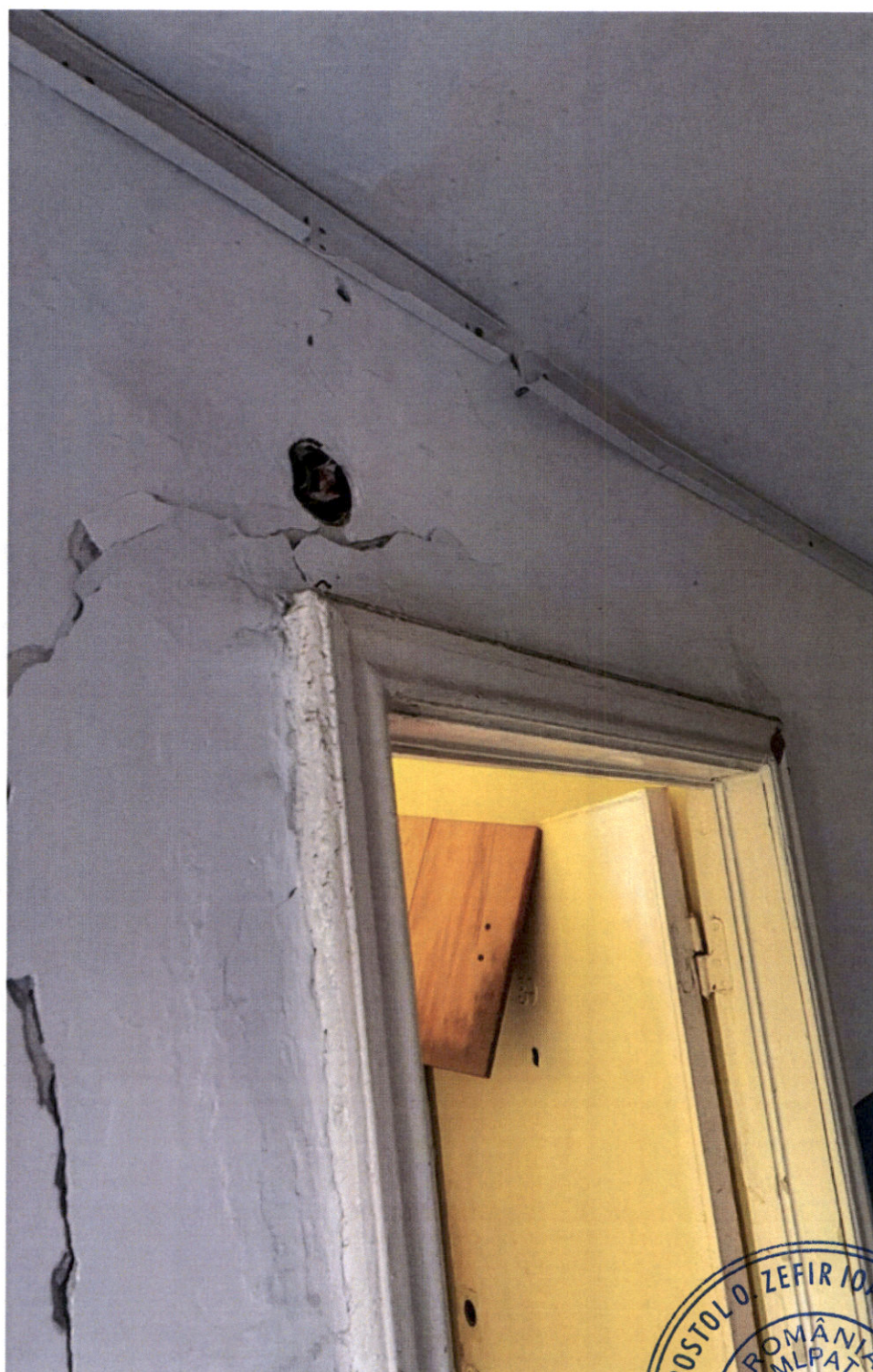
-Fisura in perete structural-
