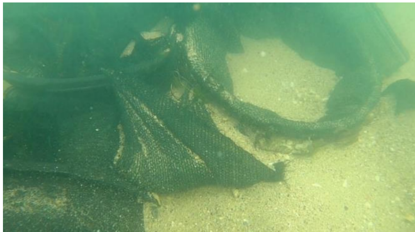
Aspect al cosurilor deteriorate
