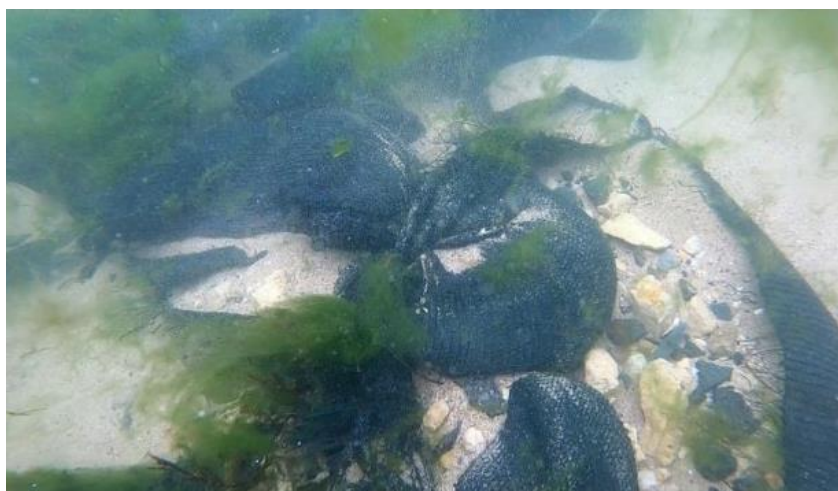
Aspect al cosurilor deteriorate
