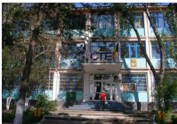
Fig. 9.15. Liceul Industrial Energetic
