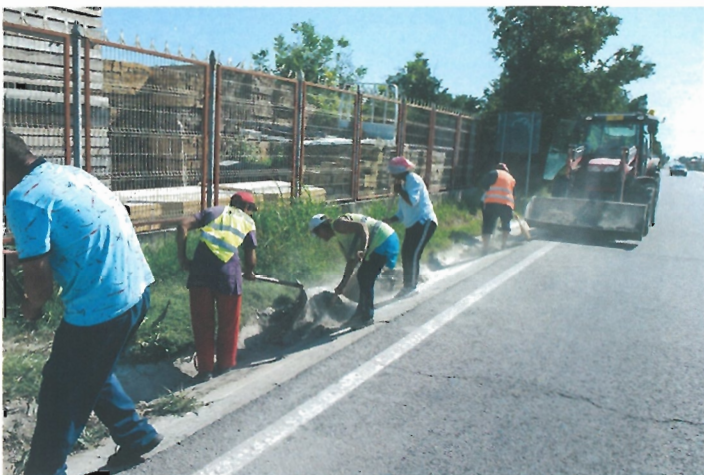
Curățare rigole prin SRL primărie / Cleaning of gutters by the Town Hall LLC
