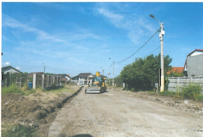
Santier drumuri / Road construction site
