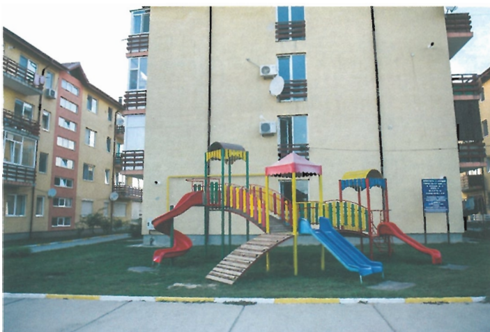
Blocuri ANL (fonduri atrase) / ANL Blocks of flats (attracted funds)
