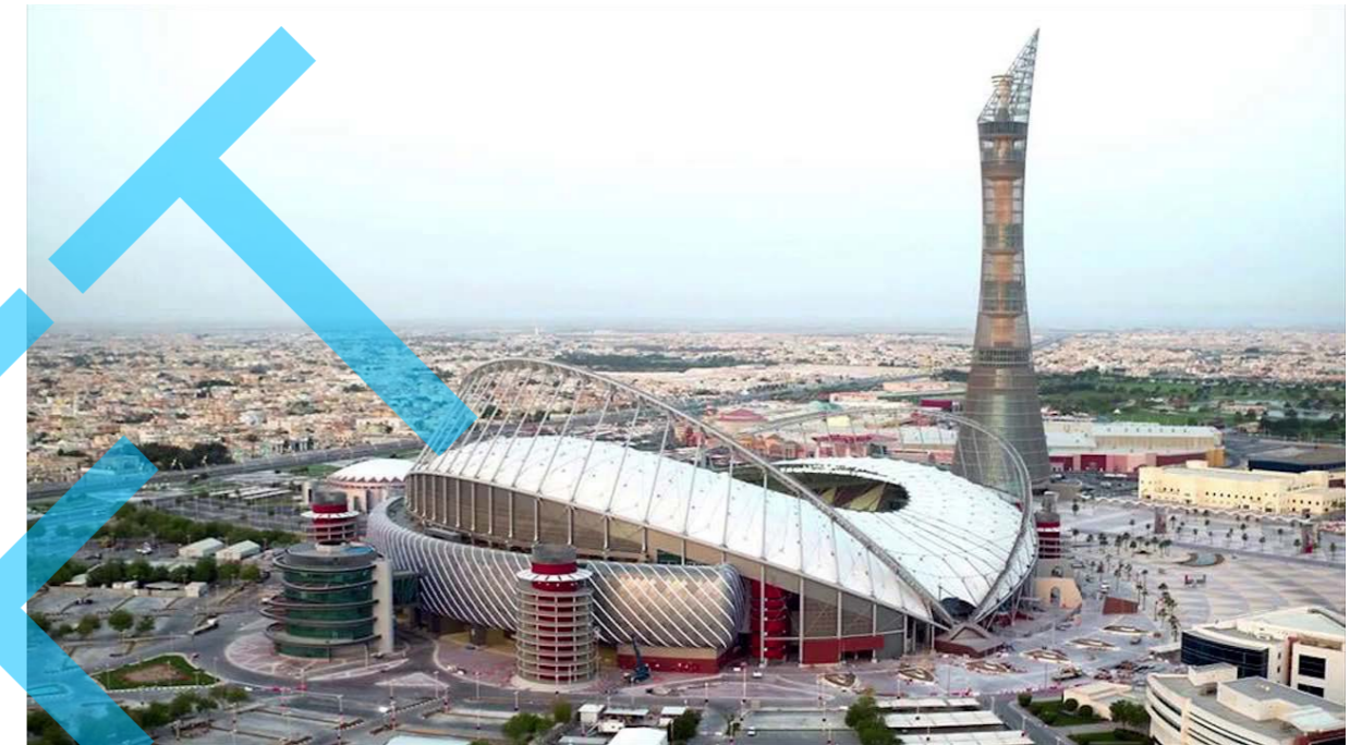
Exemplu: Khalifa International Stadium, Qatar. Sursa: timesofmalta.com
