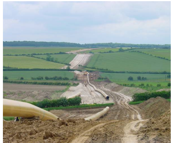
Fig. 1: Pipeline development across Cambridgeshire
